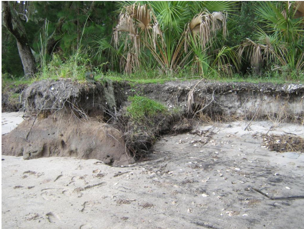
Figure 13. Brickhill bluff, erosion after heavy storm in 2007 (Courtesy John Fry, CUIS National Seashore).
