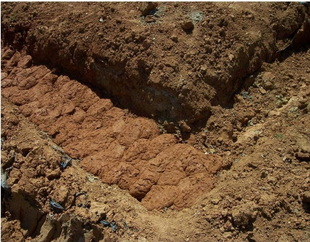
**Figure 5. One course of blinding installed over rock foundation.**
